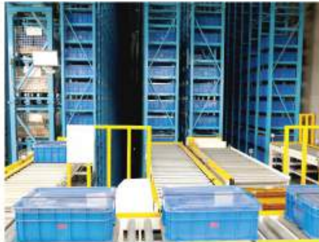
▲ Automated Storage and Retrieval System
